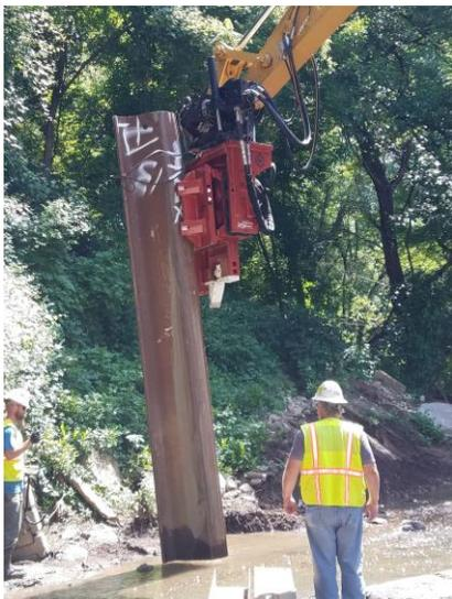
The New MKT V-8 was sent out on its first job in Louisville, KY. They are driving sheets in a drainage ditch to excavate and install a new sewer line, the sheets are short in the beginning but will be up to 30' long by the end of the project. Performance is looking good as expected, Chris Cayce and Nick Whisler will be making multiple trips to monitor the performance. We are very excited about the potential of this new design and will keep you updated as things progress.
